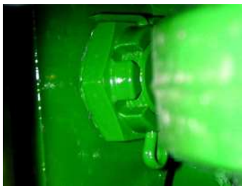
Fig. 68 Nut – Crawler belts NOT tightened
