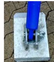
Fig. 14 Foot plate mounted and secured
