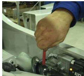
Fig. 36a ball valve emergency basket leveling.
